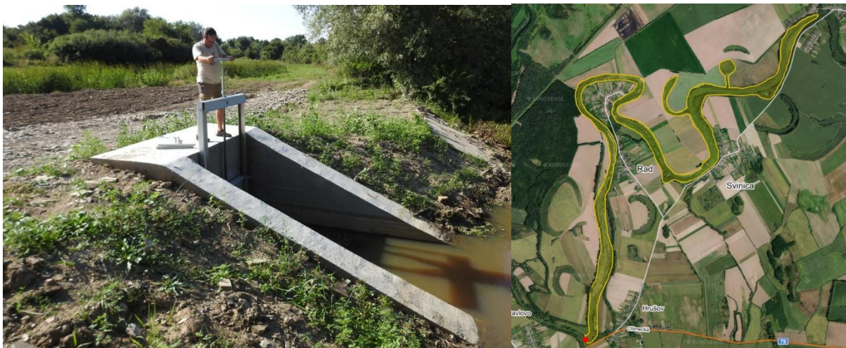
Fig. 4. Sluice gate in drainage channel and affected area by this structure
