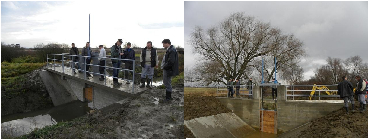
Fig. 3. Sluice gate near Iňačovce in K23 drainage channel
