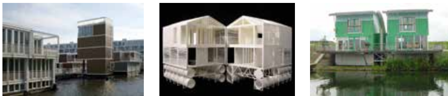
Figura 8.34 - Estruturas sobre flutuadores na Holanda (fonte: Design Ideas Daily, Factor Architecten, Florian Holzherr). http://www.inspirationgreen.com/floating-homes.html
